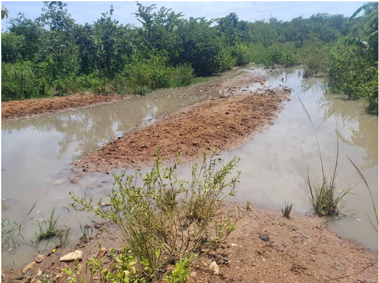
Figure 30: Water degradation through erosion and deposition
