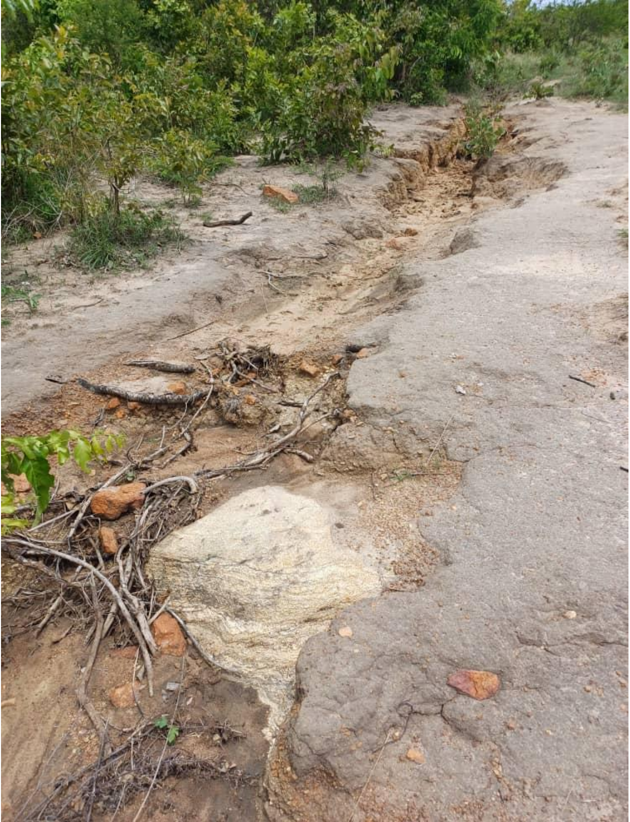
Figure 35: Gullies, a characteristic indicator of soil erosion
